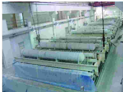
▲ 叶滤机组 Moore filter group
